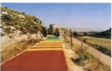
14 LINEAR PARK Architect: Marco Navarra Completed: 2001 Location: between Caltagirone and Piazza Armerina
