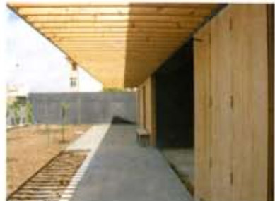
32 SINGLE FAMILY HOUSE Architects: Gianfranco Gianfriddo, Luigi Pellegrino Completed: 2004 Address: Contrada Piana, Buccheri
