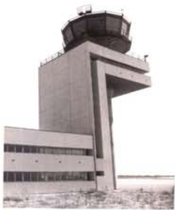
1 CONTROL TOWER Architect: Manfredi Nicoletti Completed: 1977 Address: Catania Airport
